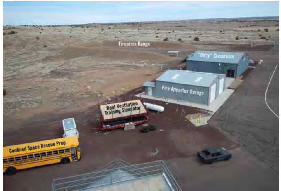
Taken from atop the 5-story Burn Tower, showing the existing classroom and area where new building and residence unit will be placed.
